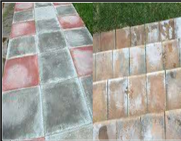
Efflorescence
