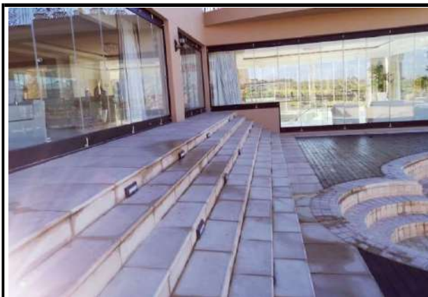
Tile Copings & Tiles on Risers
